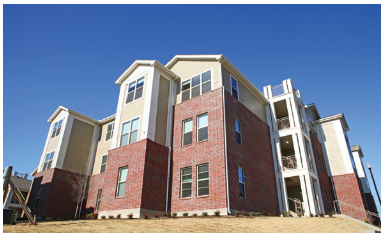
Phase one of new student housing is complete with phase two well underway. (SWBTS Photo/Adam Covington)
